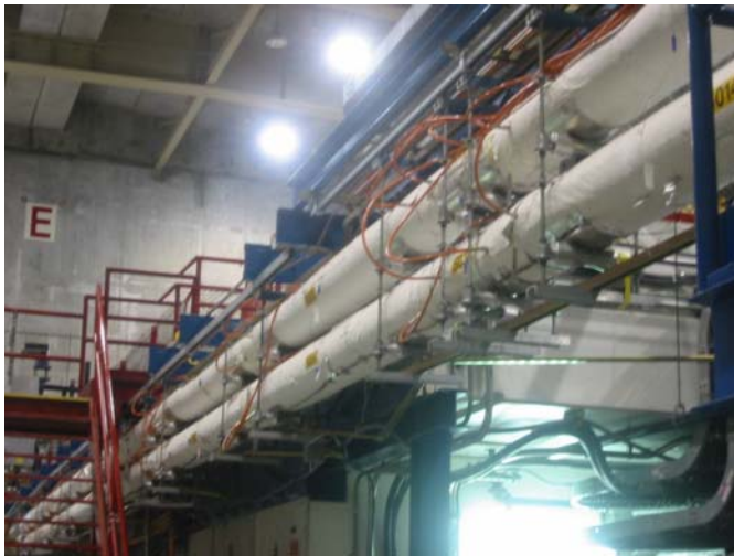
Figure 8 Large Round Waveguide Delay Line
