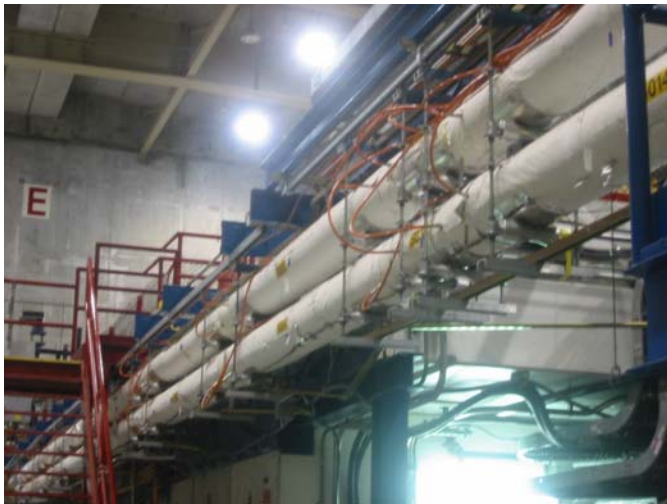
Figure 8 Large Round Waveguide Delay Line
