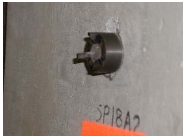
Installed Wall Monument
