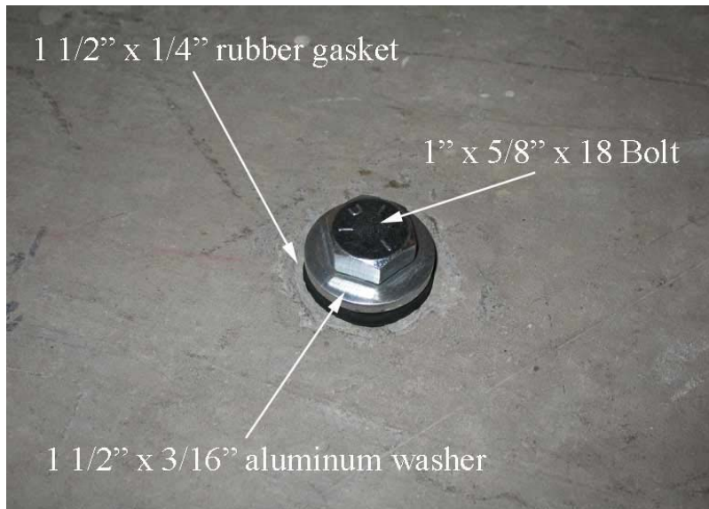
Items Inserted into Existing Floor Monument
