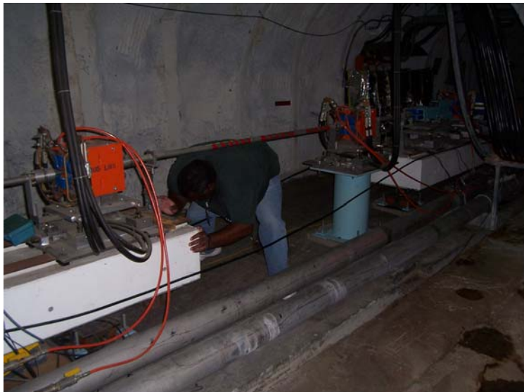
Figure 1 – Drainage Trench under Water Pipes in the Passage Way
