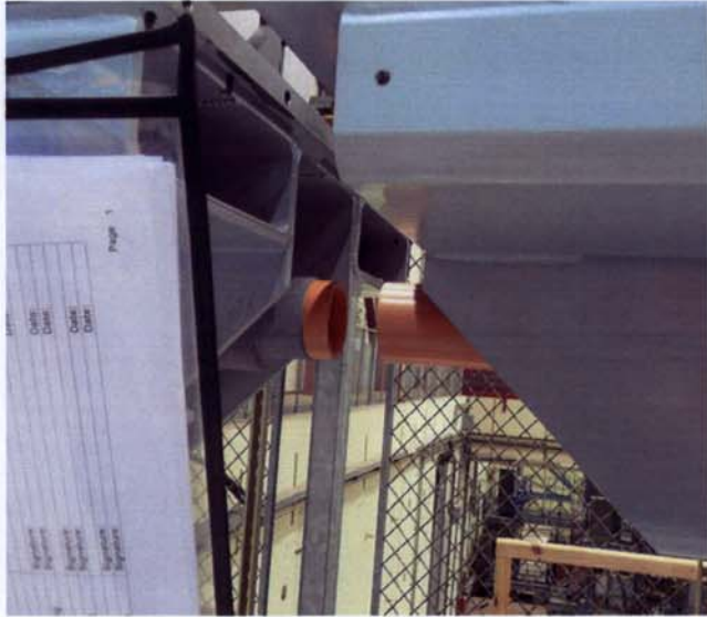
Figure 3: Before installation step
