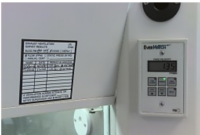
Figure 3 Quantitative Airflow Monitor and Testing Record Sticker
