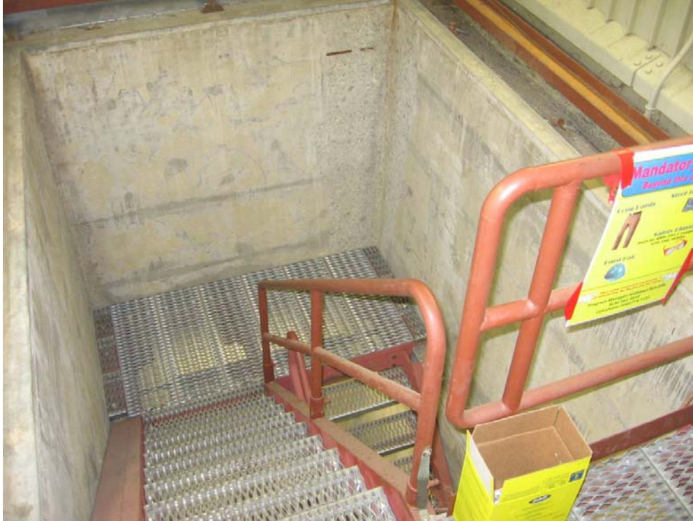
Figure 5-20. Existing stairway at Sector 24, which will be duplicated at Sector 19 for ASF users.
