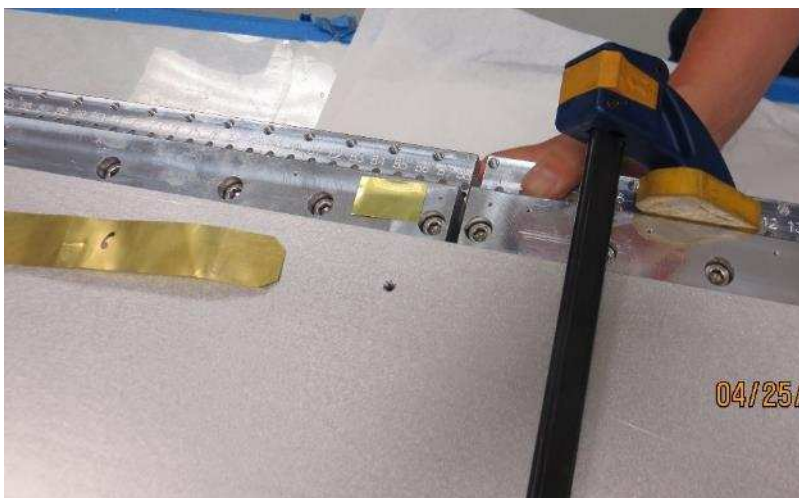
Figure 31: 0.002" and 0.006" shims ready to be placed into gap
