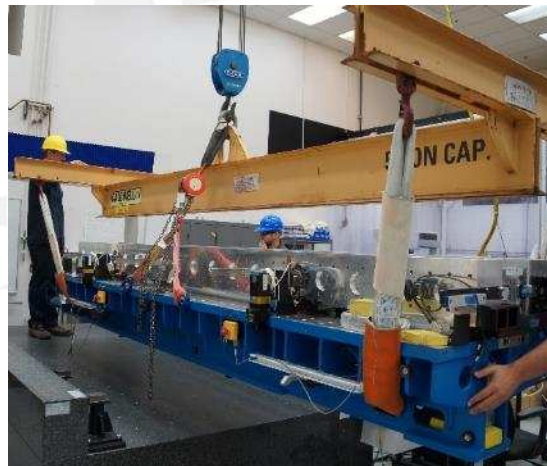
Figure 6: Lifting with H-shaped spreader bar & slings – including chainfall and lead bricks to keep level.
