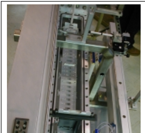
Fig. 22 Undulator segment in vessel
