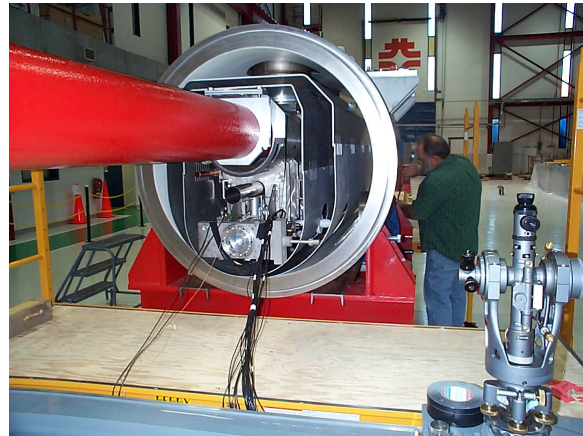
Figure 4: Insertion of coldmass mockup into vessel.
