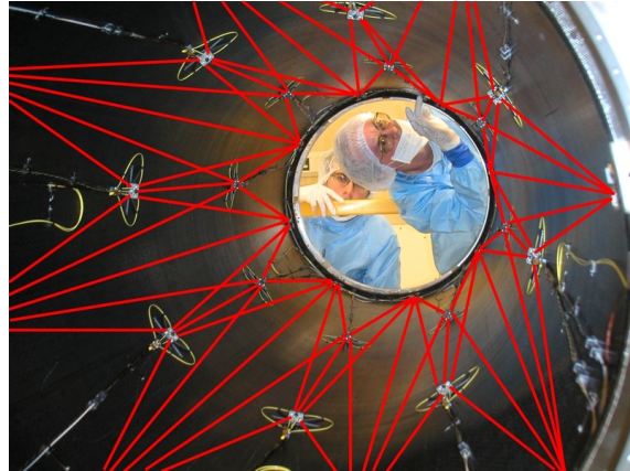
Figure 2: The FSI grid nodes installed within a support cylinder of the SemiConductor Tracker. Each grid line is an interferometric length measurement precise to < 1 \mu\text{m} .
