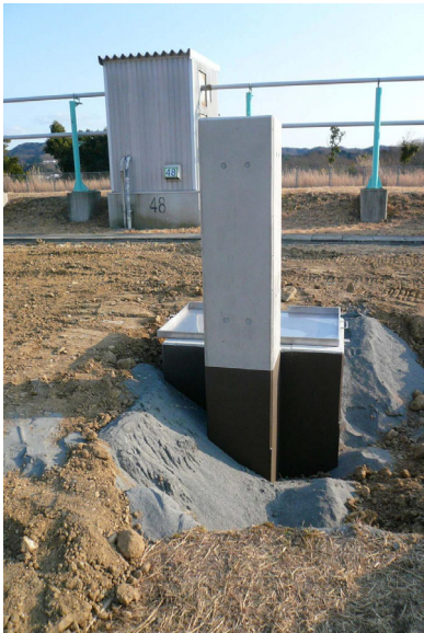
Fig.3 The HLS pit, lower part of monument, is buried underground.
