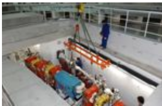
Figure.10: Crane of front-end
