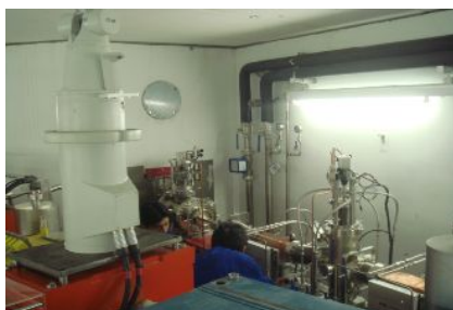
Figure.11: Installation of front-end
