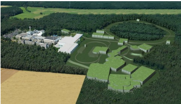
Figure 1: Aerial view of GSI with photo composition showing FAIR
