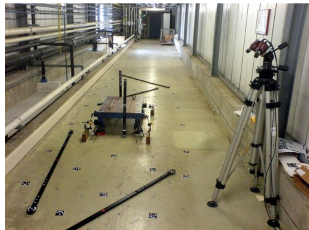
Figure 8: Test installation. On the right hand side the two cameras are mounted at 130 cm height on a tripod. Coded and uncoded targets as well as six scale bars are placed on the floor. In the center part the table can be seen which is used to simulate a misaligned magnet.
