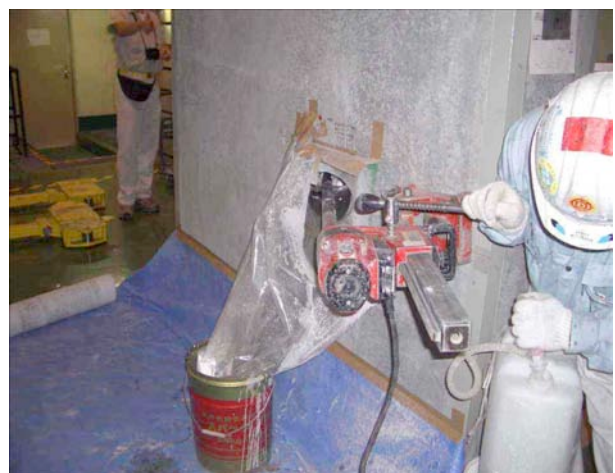
Figure 8: Drilling a hole through the concrete block.
