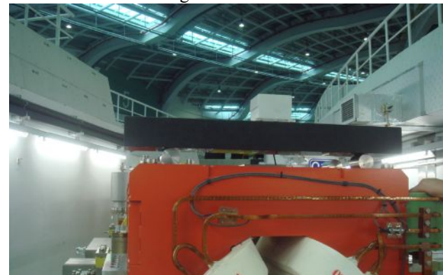
Figure.14 Inclinometer check of storage ring
