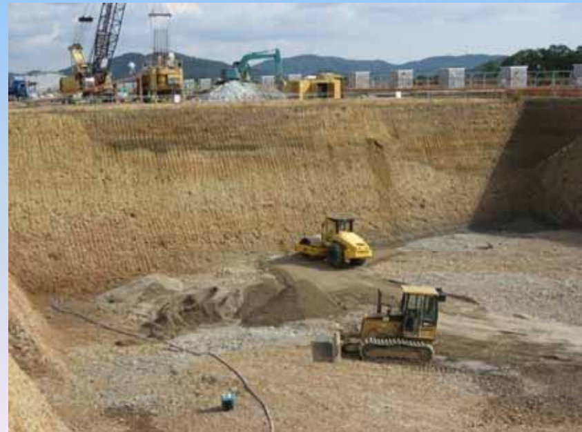
Paving with crusher stone
