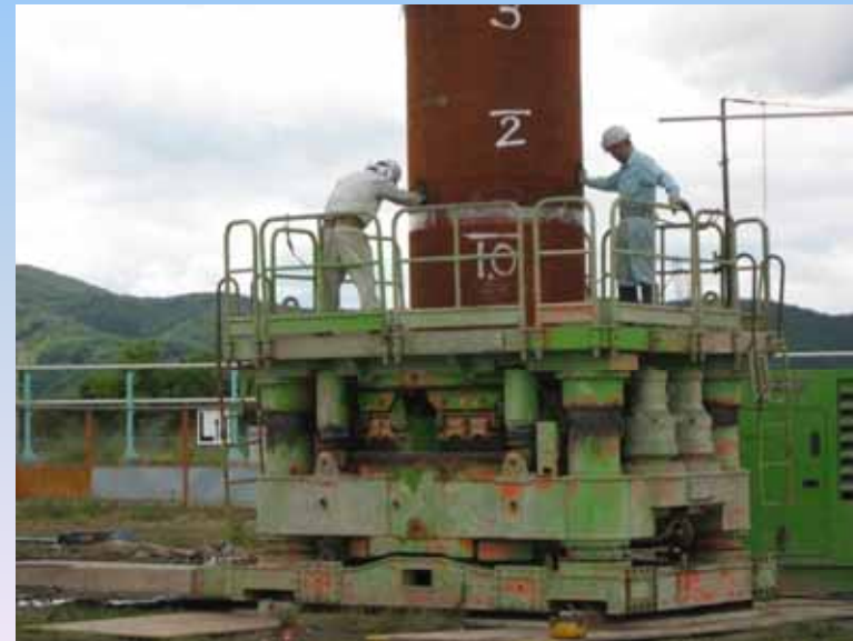
Press Fitting of the Pillar Casing
