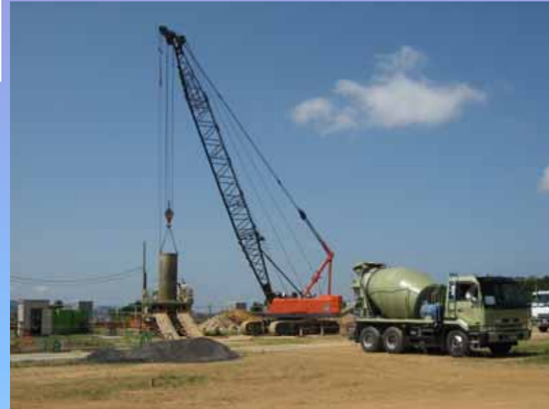
Basement Pillar Construction
