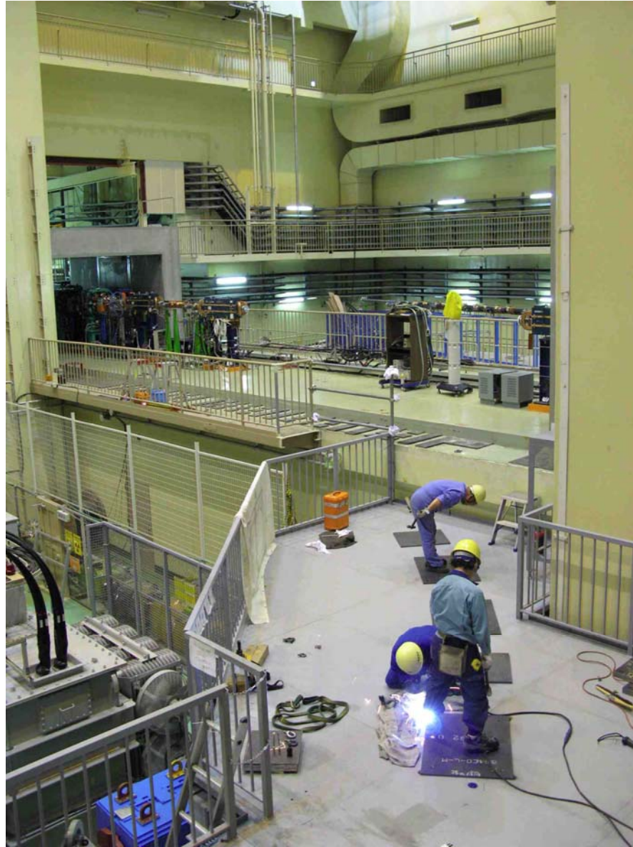
Welding iron plates on the stage.
