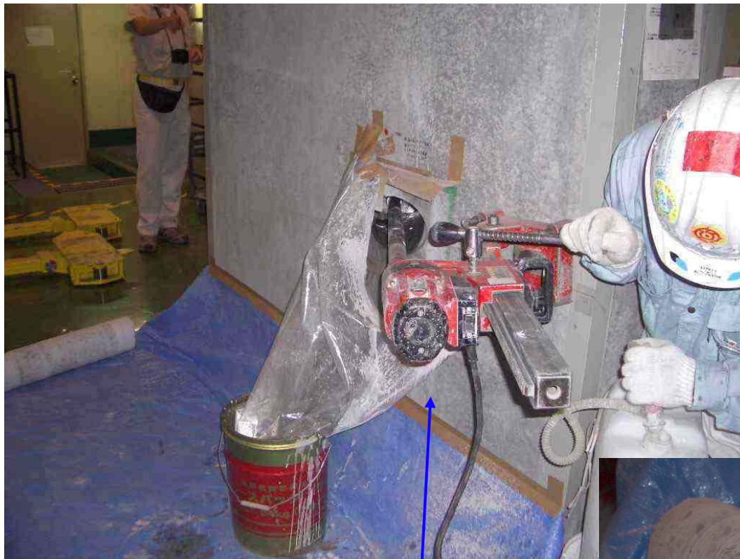
Drilling a hole in the concrete block shield.
