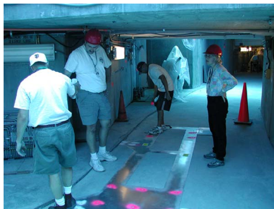
Fig. 10 Marking Anchor Hole Locations
