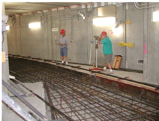
Fig. 9 Surveying Screed Rails
