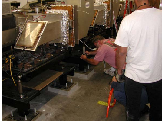
Fig. 12 Aligning the RF Cavities
