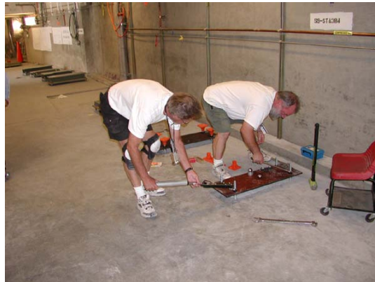
Fig. 11 Setting Support Plates
